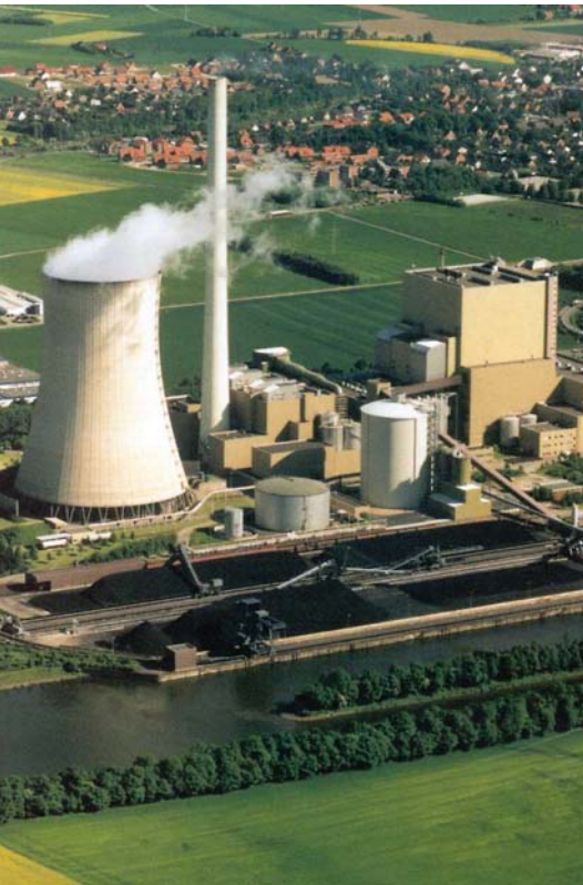
In the mid eighties a hard coal-fired unit was built north of the German town Porta Westfalica. At present, this unit has the highest capacity in Europe at 865 Megawatt.
