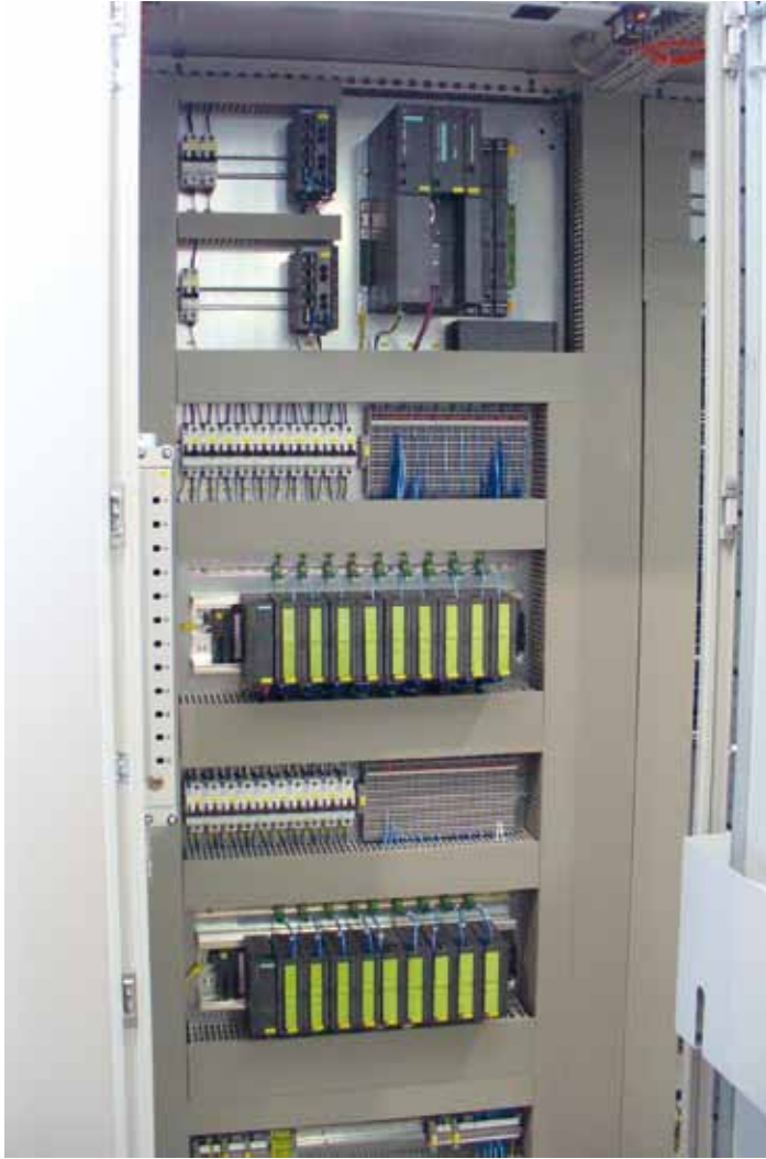
Schrank CPU und E-A-Ebene CPU cabinet and I/O rack
